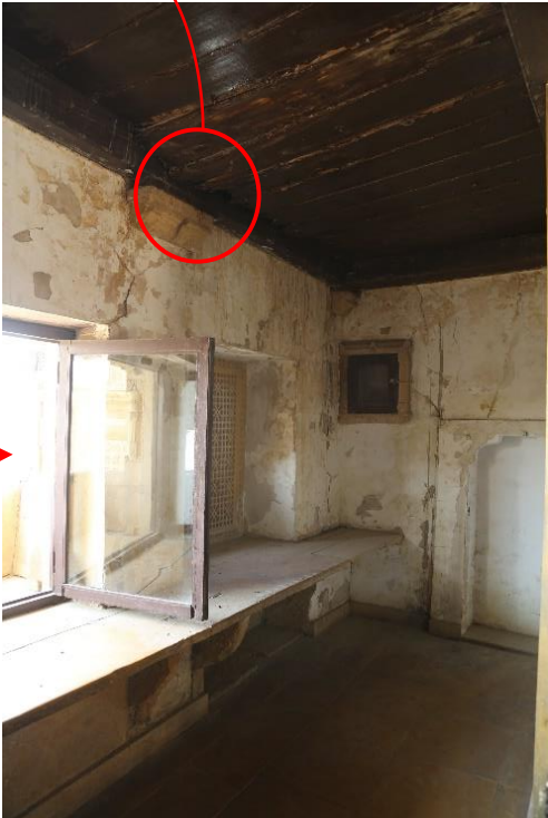
Deteriorated wall and damaged wooden ceiling supports
