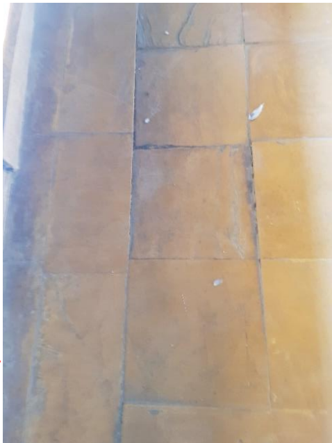
Collapsing/sinking areas in floor
