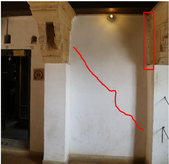
Separation of bracket and cracks on wall
