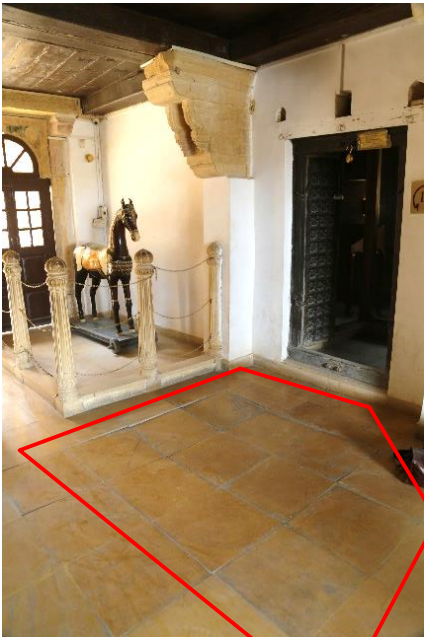
Collapsing/sinking areas in floor
